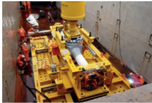
Subsea Riser Positioning
